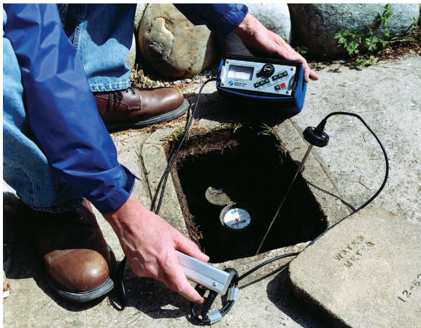
Figure 4-8 Leak Survey at a Meter
